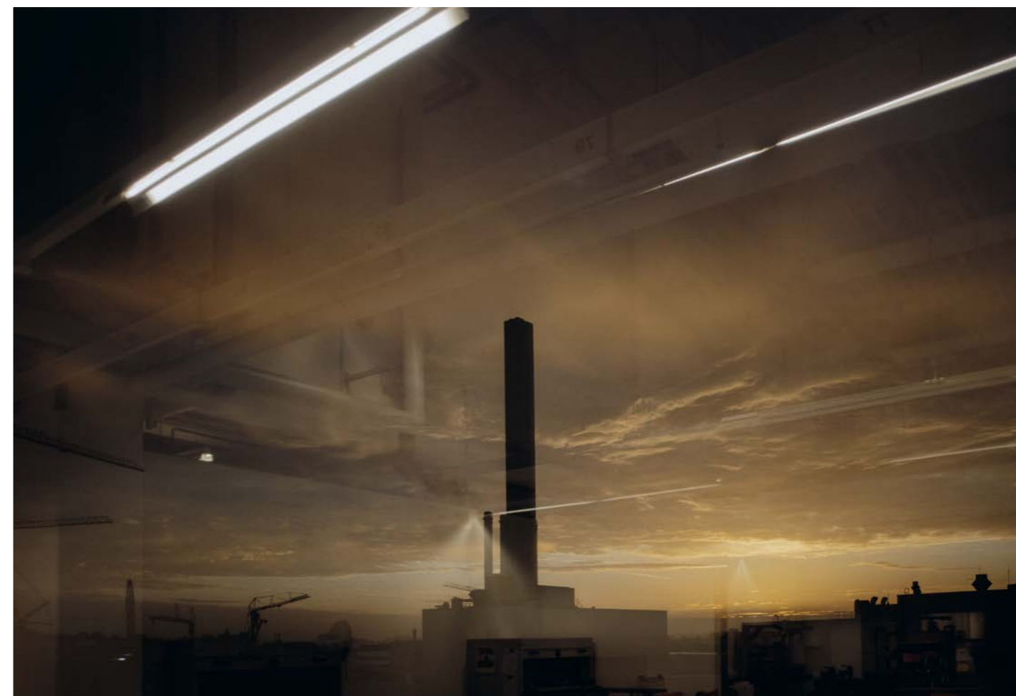
Dawn: Around a billion euros are flowing into the most ambitious project in Porsche's company history, a new plant for electric vehicles at the company headquarters in Zuffenhausen – a new age with new technologies for 1,200 jobs.
